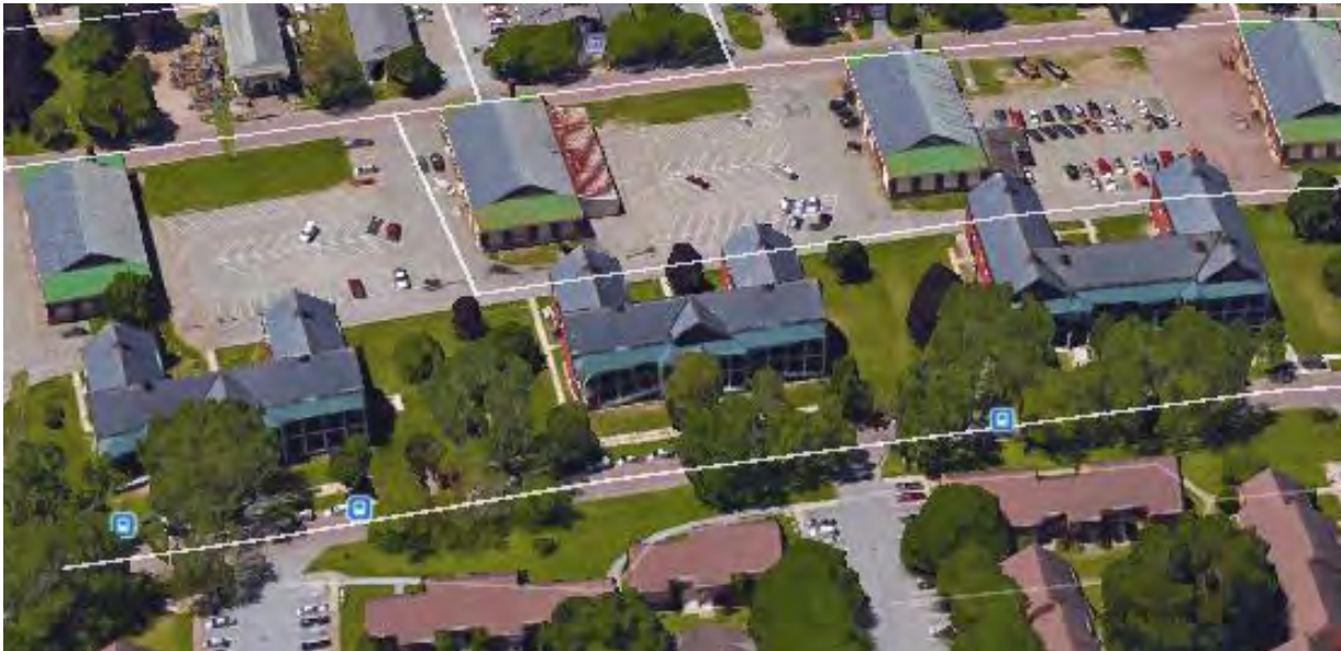
Repurposing College Dormitories for Affordable Rental Housing
